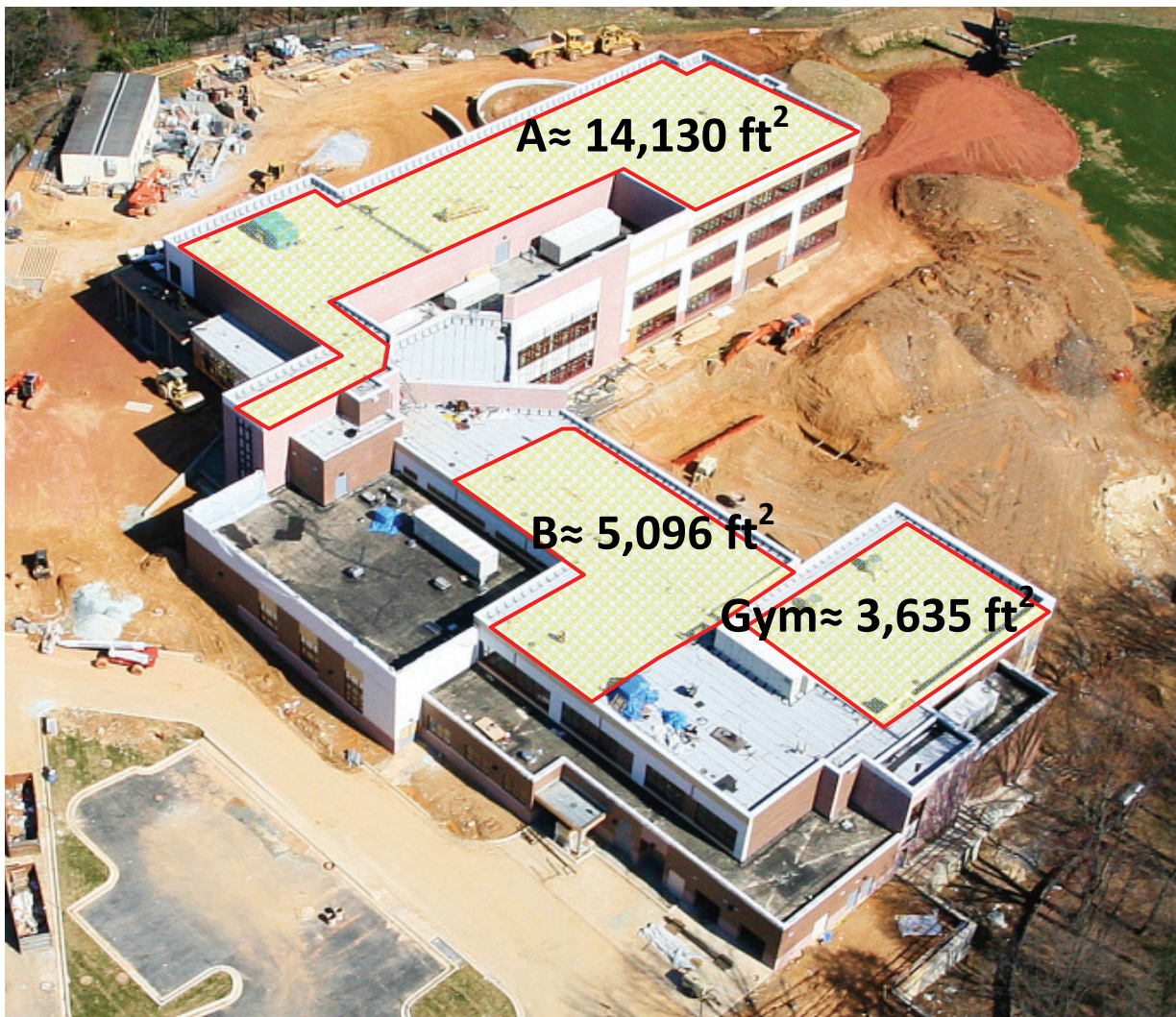
Figure 26 - Location of Solar Panels on Roof
